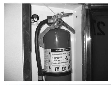
Figure 4.37 Type A-B-C fire extinguisher
