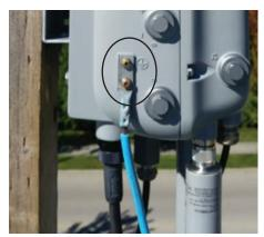
Figure 4-8 An Outdoor Access Point with Electrical Grounding (Photo Credit: Ian Procvk)
